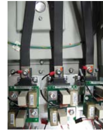
R, S, T Bus Bars at SCR
