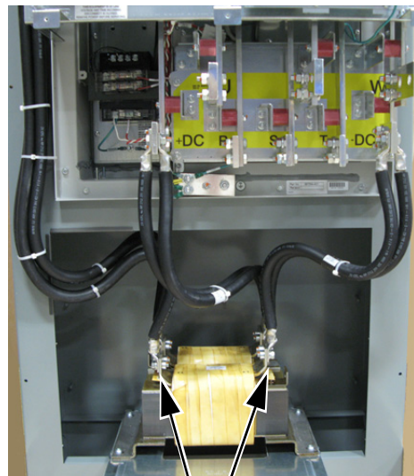
+DC (Back/L2 Connector) +DC (Back/L1 Connector) -DC (Front/L3 Connector) -DC (Front/L4 Connector) DC Choke Connectors
